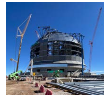
The ELT under construction by ESO; the primary mirror will have a diameter of 39m
